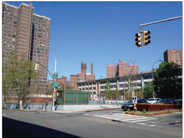
View southwest from Montgomery Street and South Street 8
