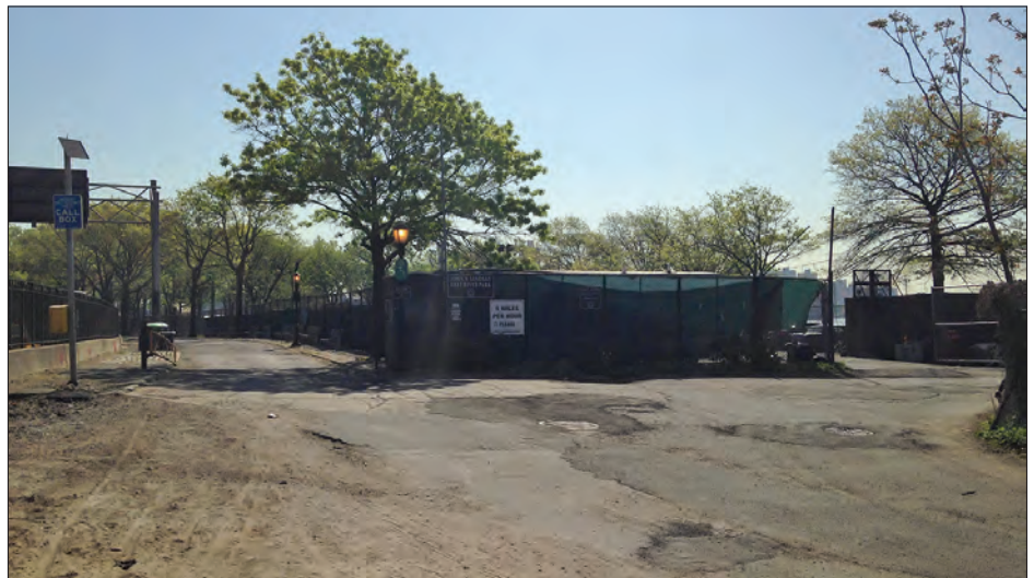
View of Pier 42 apron / East River Park portion of project site 3
