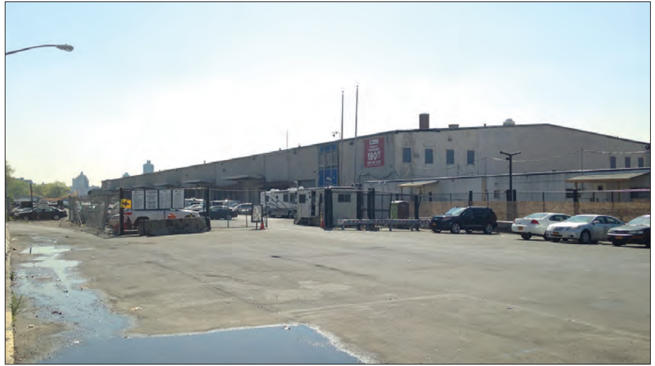
View of Pier 42 pier shed and apron 1
