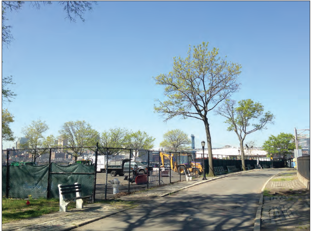
View of the East River Park portion of the Project Site facing southwest 3
