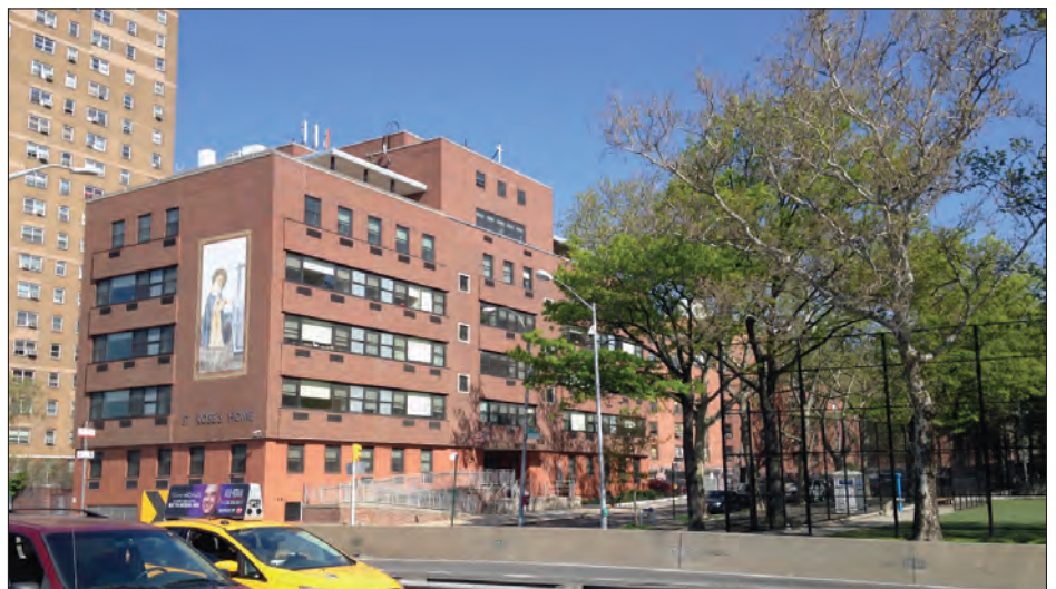
View inland from project site 6
