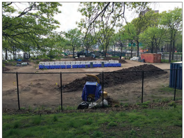
East River Park area adjacent to project site 12
